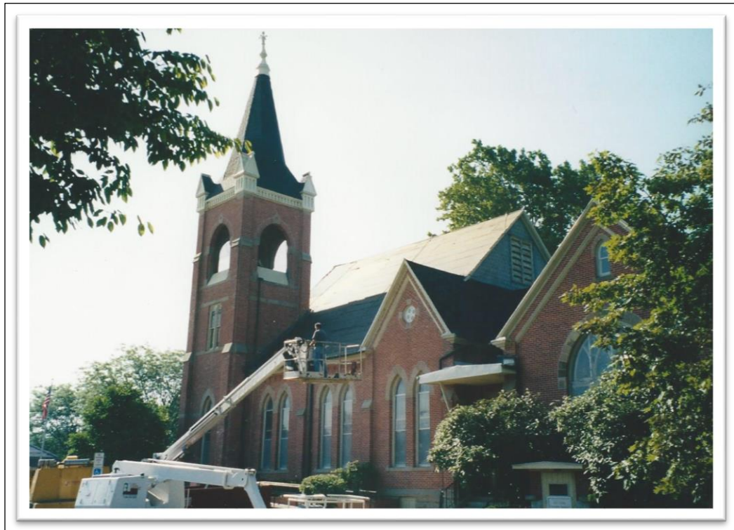
The Ada Presbyterian Church gets a new roof in 2002.
